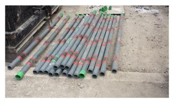
The Drilling for the sleeve installation has been made with temporary casing removed only after the PVC sleeve installation sealing the annular space around the PVC sleeve with a plastic mix cement-bentonite.
