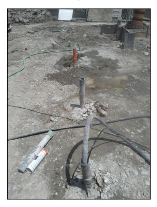
The grouting operation were made in ascending sequence valve by valve and sleeve by sleeve until close the perimeter around the secant caisson wall, after reach the refusal criteria for the permeation grouting operation.
