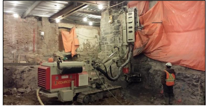
Comacchio MC-600 drilling vertical dowels inside the building for foundation underpinning.
