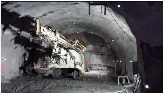
PG-115 drilling the umbrella of micropiles inside the tunnel.
