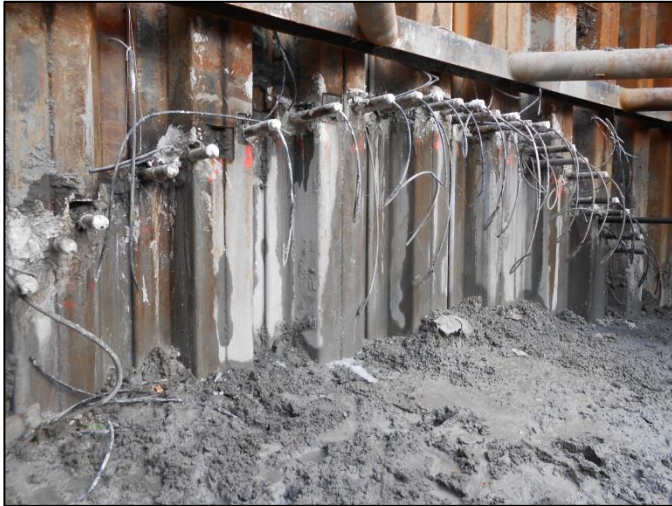
Umbrella of Micropiles at East Portal.
