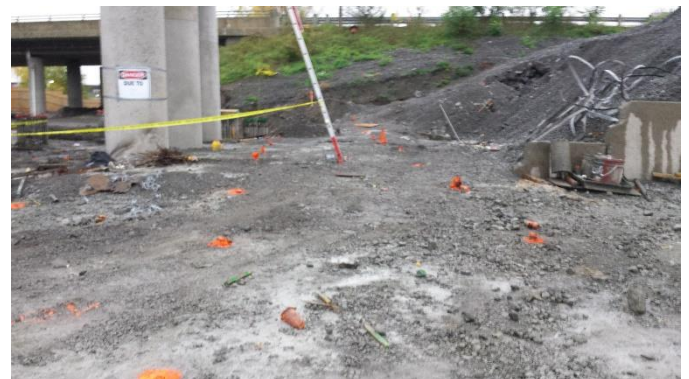
Figure 2. Secondary injection system grid installed.
