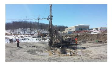
After the approval of Site Canada design, with the result of the production micropiles, the installation of the soil anchors takes place between January and December 2016.
