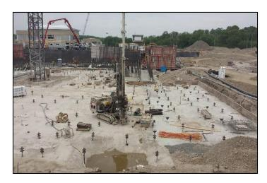
Before the start of the production soil anchors and to confirm the design solution, a campaign of verification test take place in three sacrificial soil anchors tested at 200% the Design Load.
