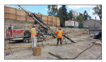
The assembly of the tiebacks has been made on the job site to deal easily with any change of dimensions of the free or bond length if there is any change in the Geotechnical conditions during the drilling operation.
