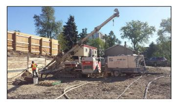
The tie-backs are made with 4 strands of 0.6" diameter ASTM 1860 Mpa steel grade to resist a pull-out load of 600 kN applied with a Multi-strand Jack.
