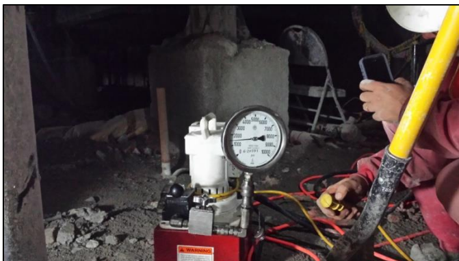
Pull out Performance test of DSI DCP Shear Wall Rock Anchor.
