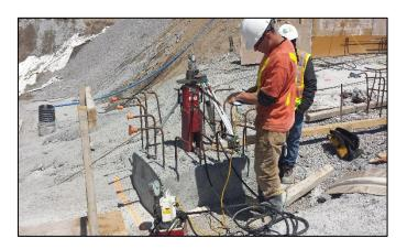
After this successful test the production soil anchors started and 348 units has been installed between October and December 2015.
